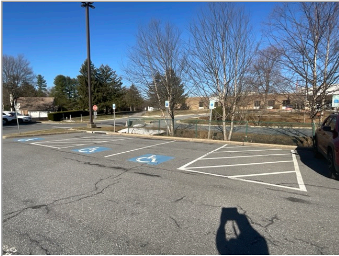
OVERVIEW OF ACCESSIBLE PARKING AREA
