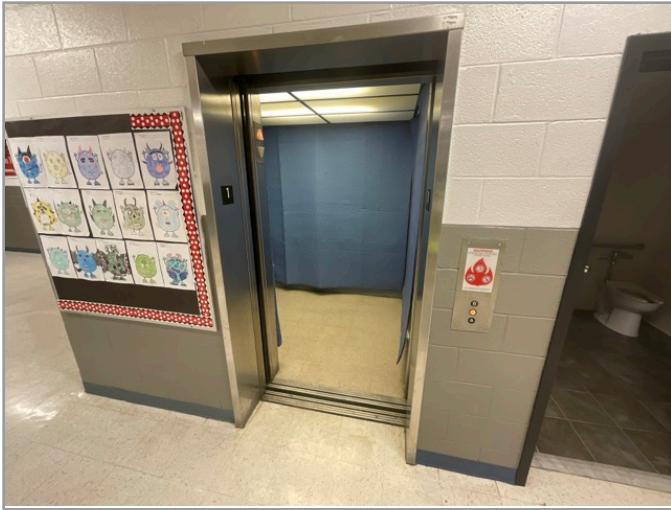
LOBBY LOOKING AT CABS
